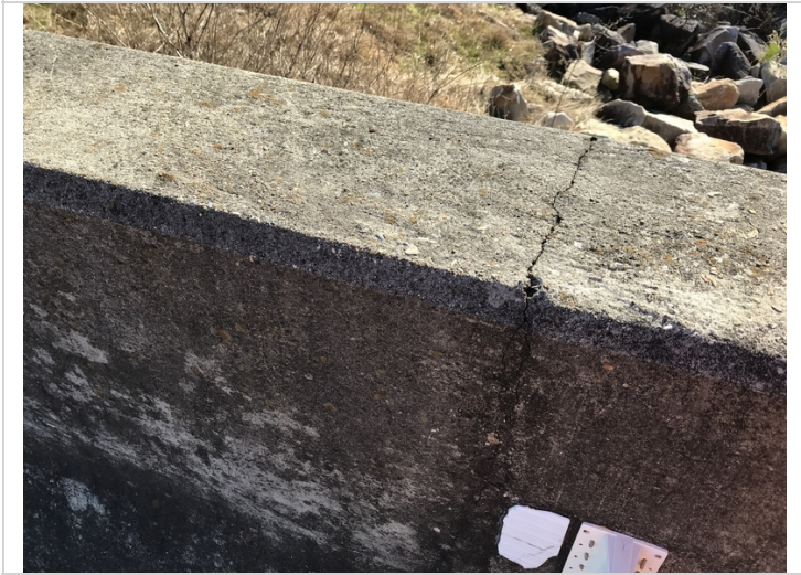
Cracking in the parapet wall
